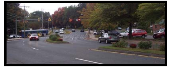
A center median, like the one above on Route 159, could be provided along sections of Route 305 in conjunction with other improvements to help preserve residential character while benefiting overall corridor safety.
