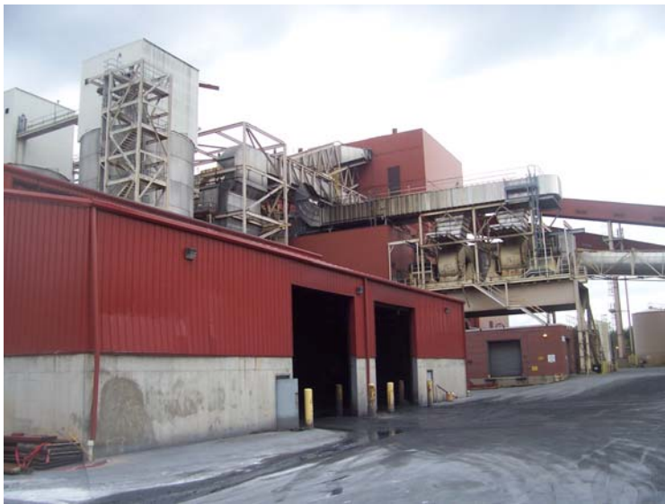
Figure 2-2 Mid-Conn Project WTE Facility
