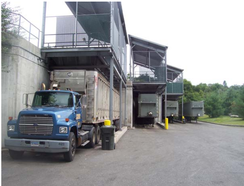
Figure 2-4 Mid-Conn Project Essex Transfer Station
