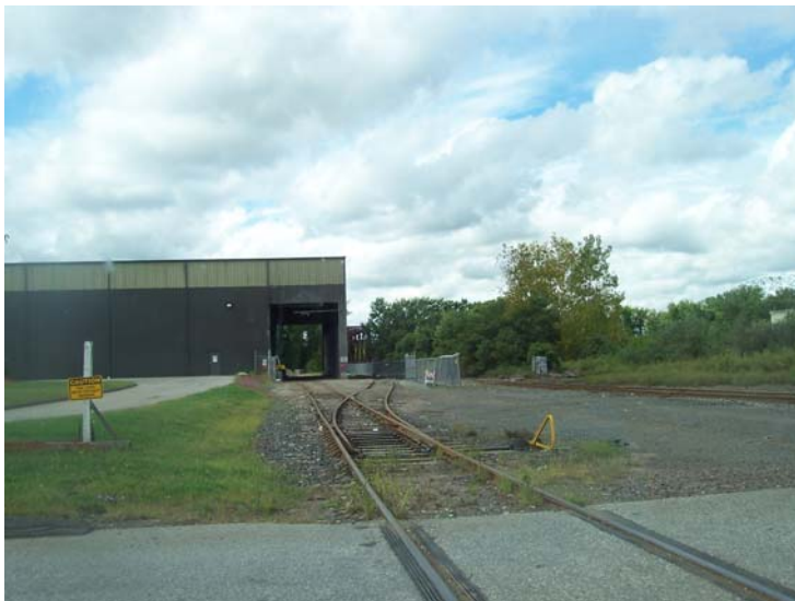
Figure 2-5 Airport Road Transload Facility
