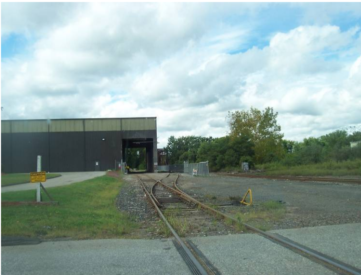
Figure 2-5 Airport Road Transload Facility
