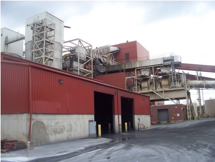
Figure 2-2 Mid-Conn Project WTE Facility
